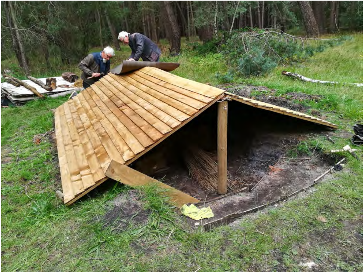
Fig.31. The shelter for the winter of 2022-3.
