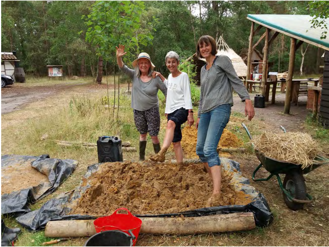
Fig.7. Puddling the brickearth with straw
