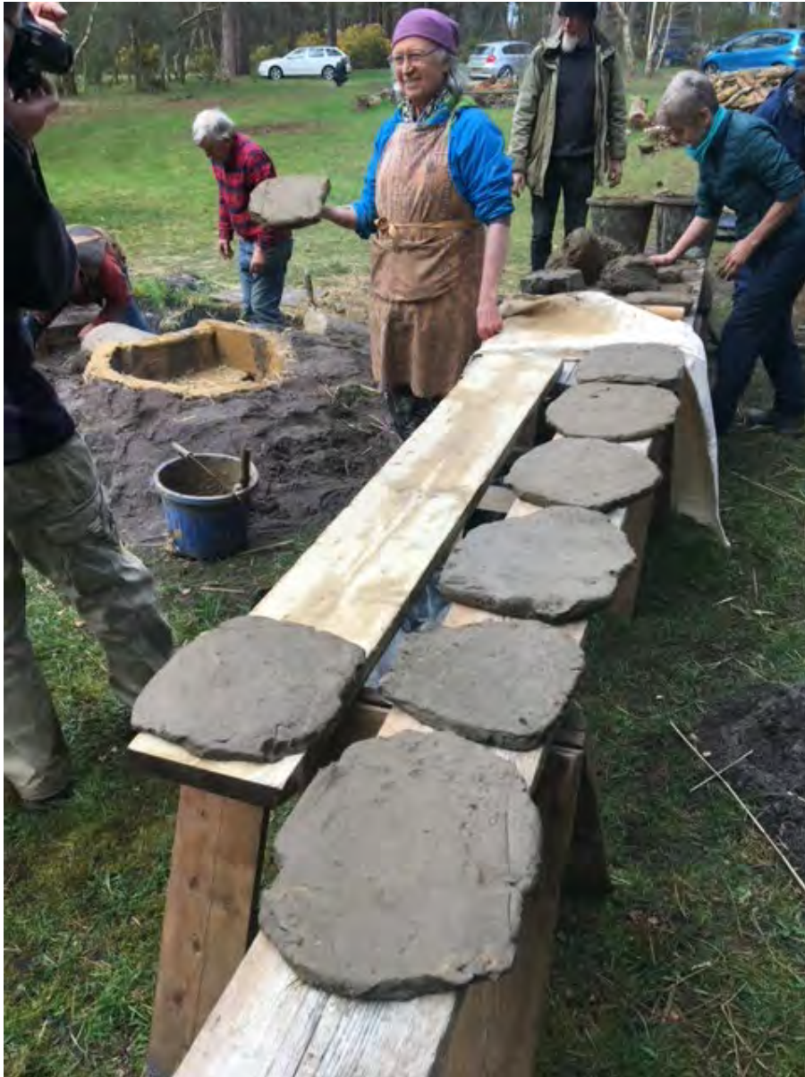
Fig.16. Making slabs of London Clay to construct the kiln dome
