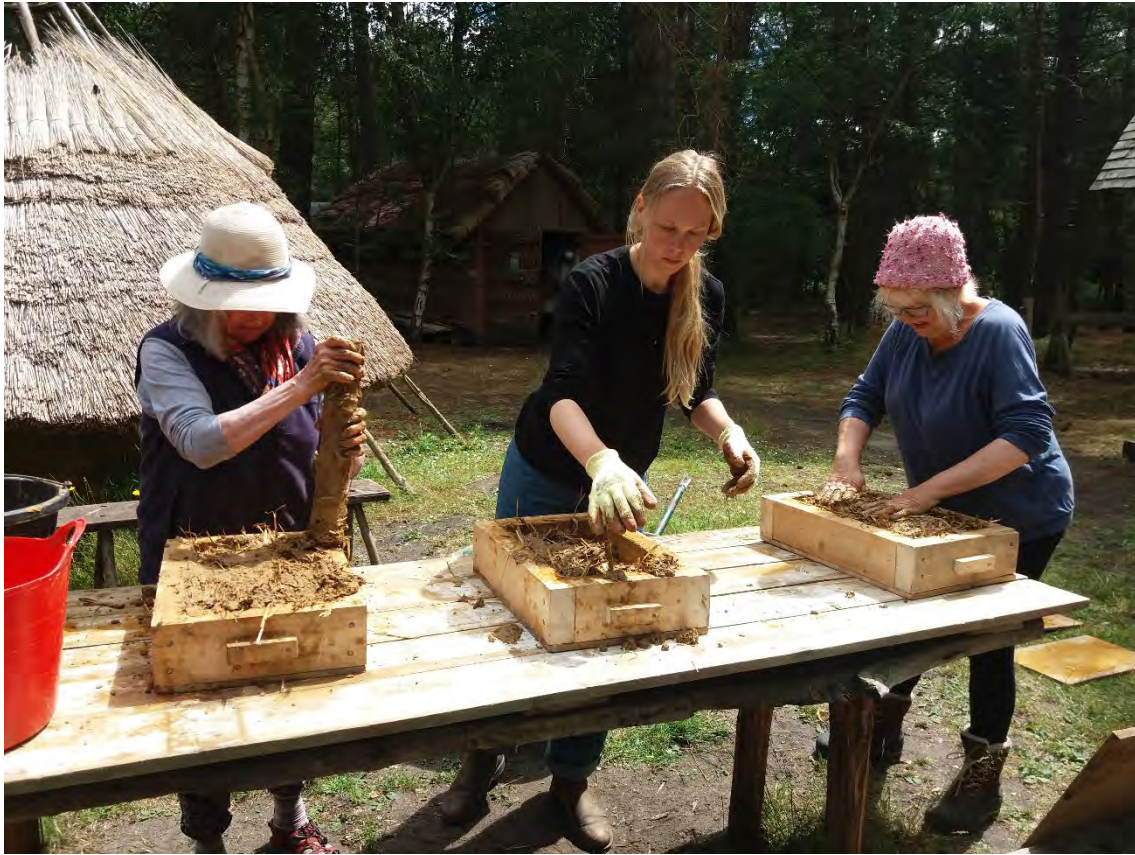
Fig.8. Packing the cob into wooden moulds.
