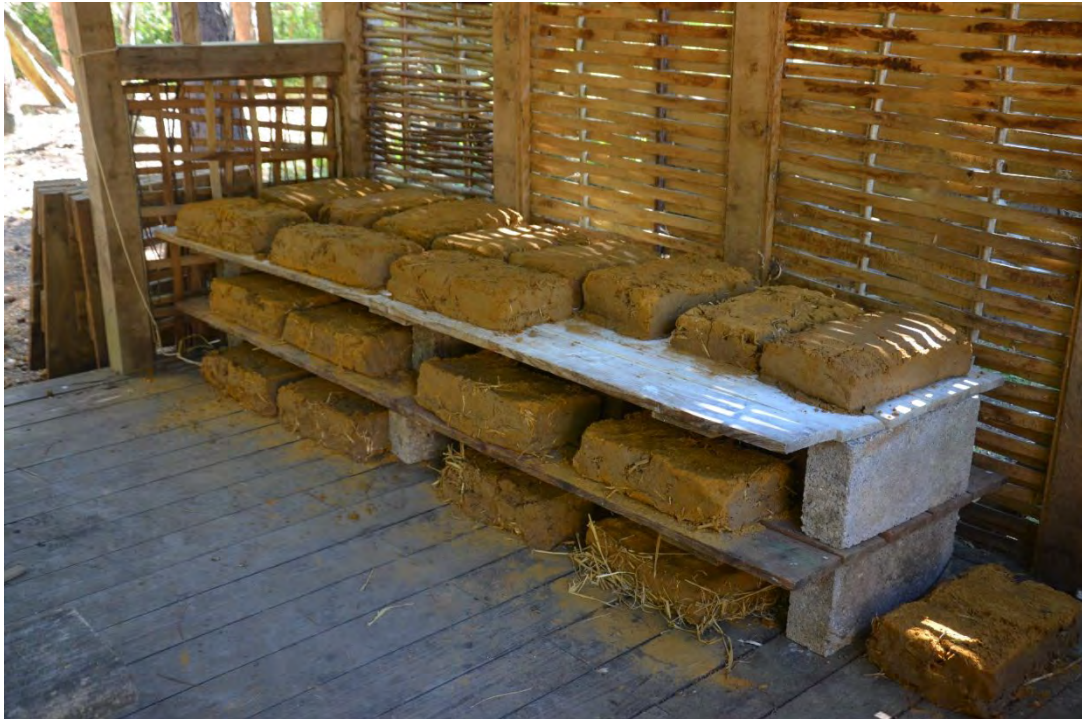
Fig.10. Blocks laid out to dry.
