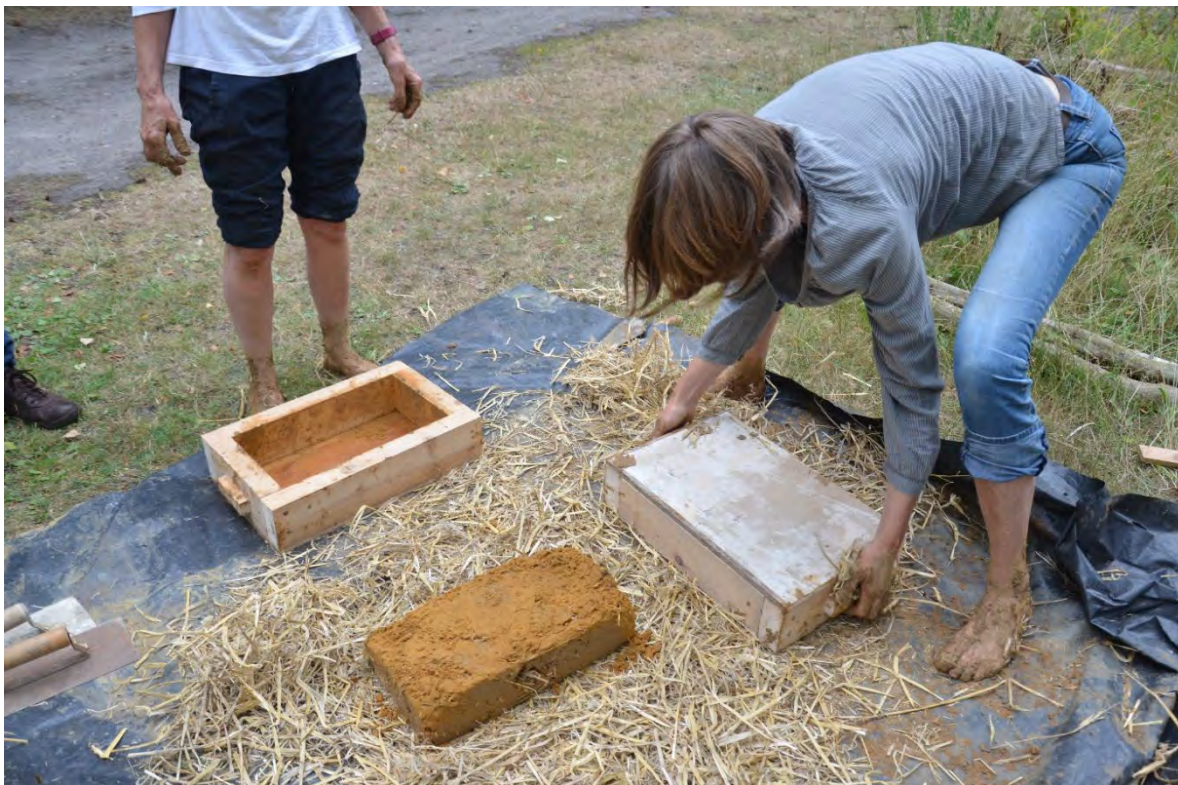
Fig.9. Turning out the cob blocks
