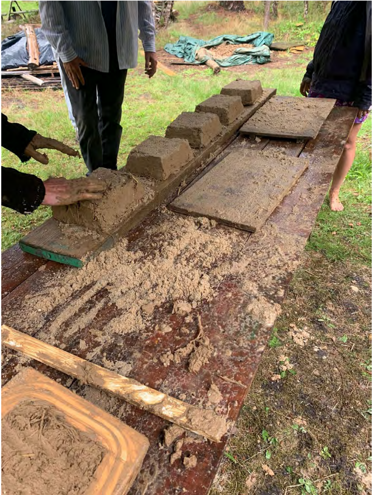
Fig.22.Making the tapered blocks to raise the kiln oven walls one course
