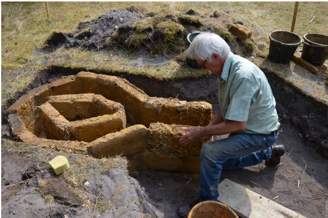
Fig.11. Building the walls of the kiln
