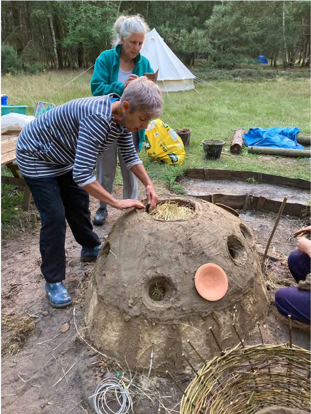
Fig.25. The dome awaiting the pre-made cap and showing the air vents
