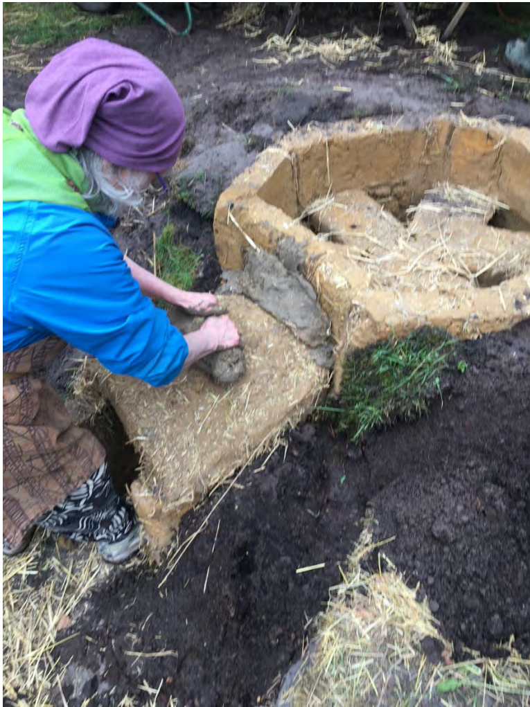
Fig.13. A further course of wall oven and the flue arch added.
