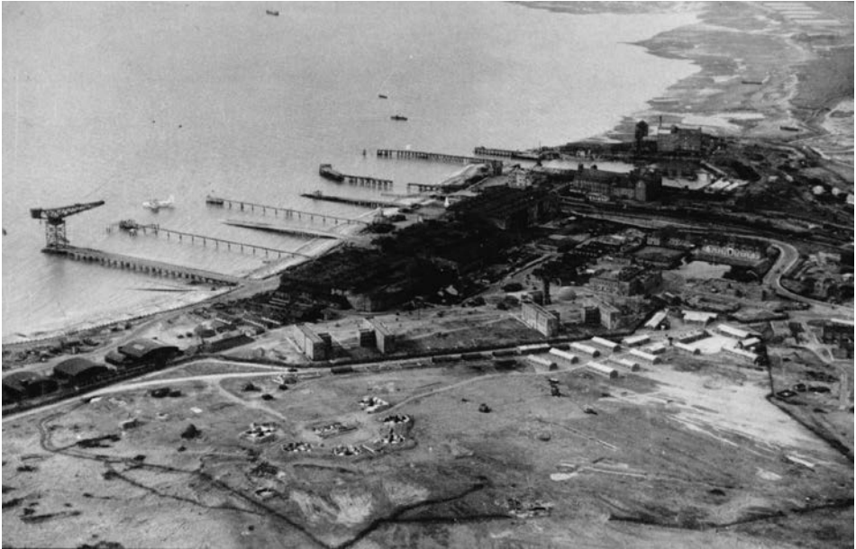
Figure 23. Early post-war photograph of Felixstowe docks, which gives an impression of the wartime infrastructure, now for the most part the modern container port. In the foreground the remains of a heavy anti-aircraft battery can be seen, while the group of buildings in the centre are Royal Navy and Royal Air Force facilities, including barracks and maintenance sheds. (Ipswich Record Office)
