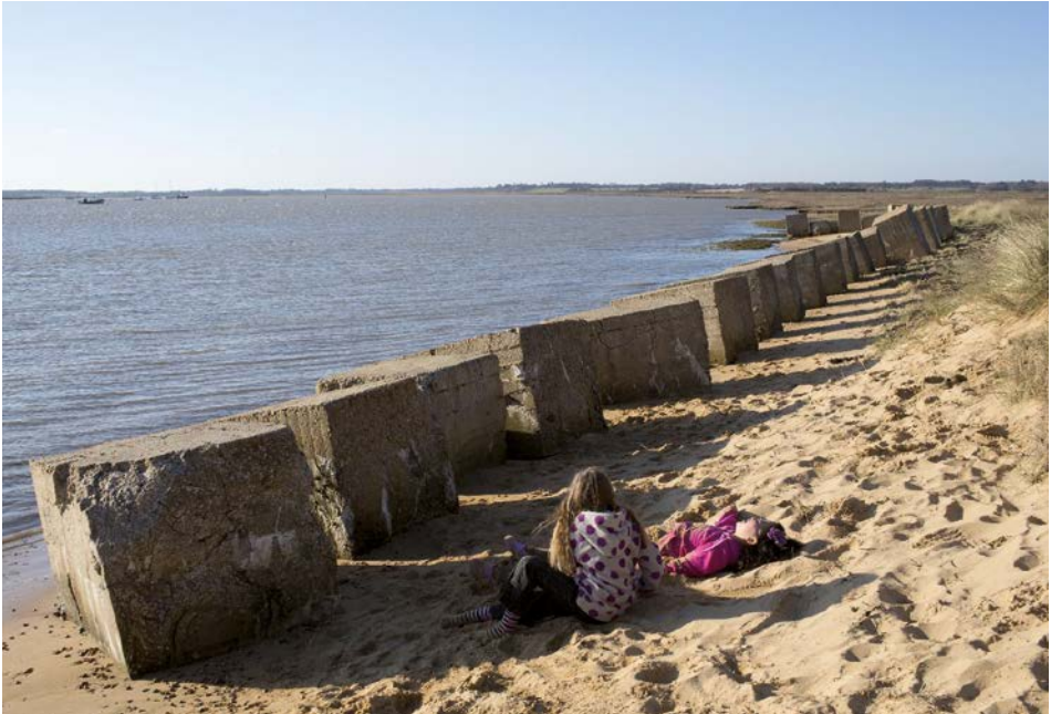
Figure 20. Line of anti-tank blocks at the mouth of the Deben at Bawdsey Point. As well as being part of the anti-invasion defences, these blocks helped to protect the southern part of Bawdsey Radar Station. (Stefan Dewickere)
